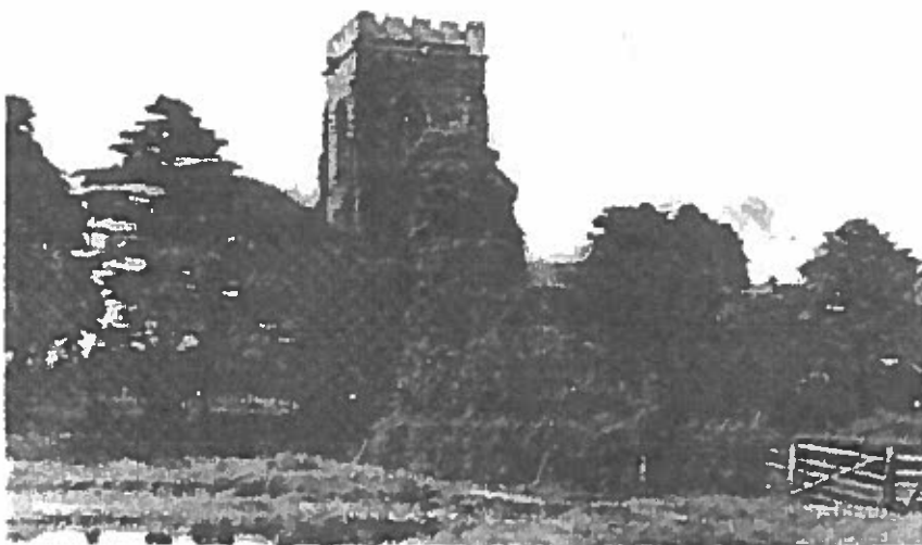
Another View of the Church Tower.
