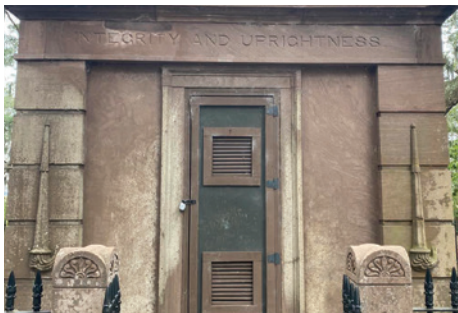
This temporary door has been removed.
