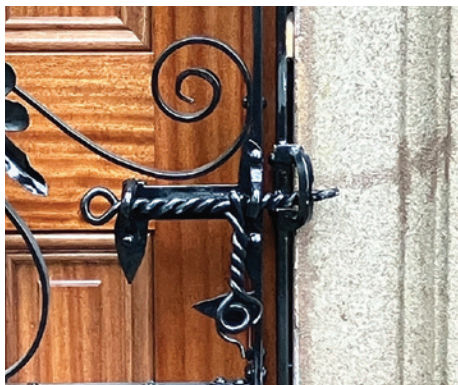
Gate hardware detail.
