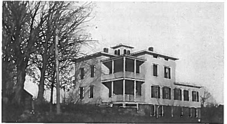
HOUSE NO. 3 ON HOLCOMB HILL, NEW HARTFORD
