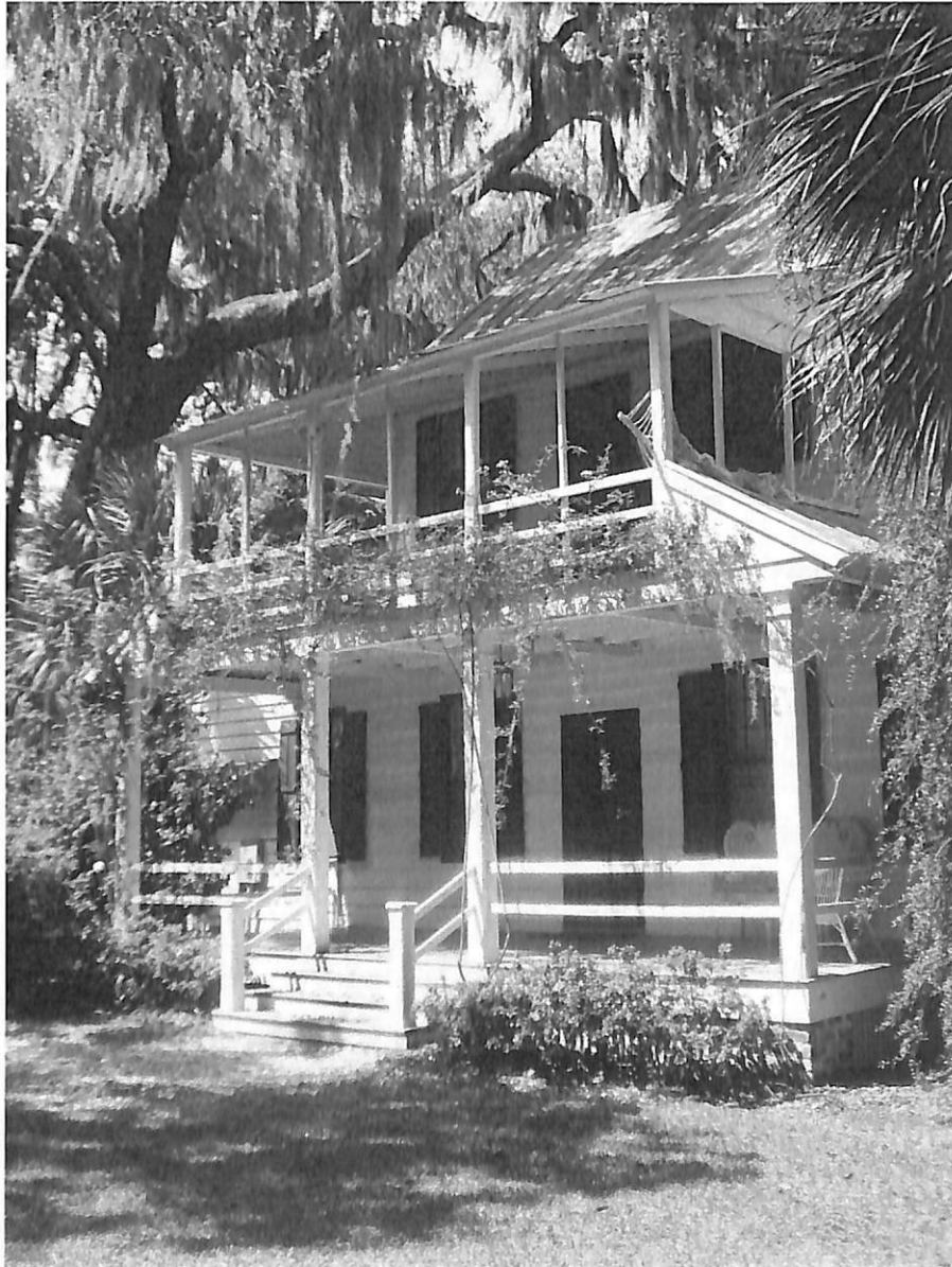
Card House, Bluffton, SC
